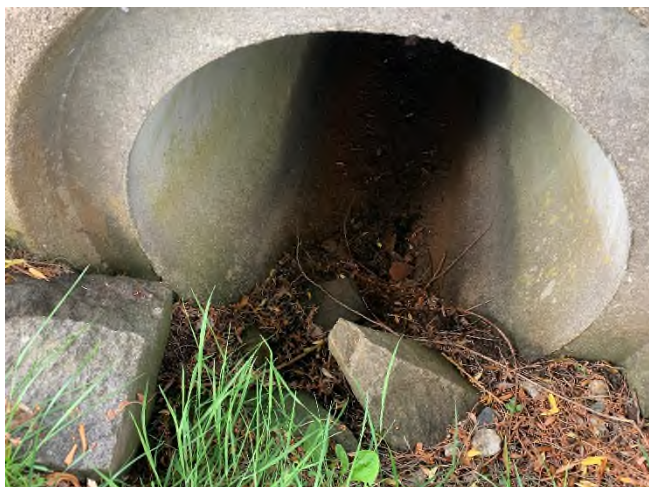
64 Gundalow - 2 (Drainage Course)
