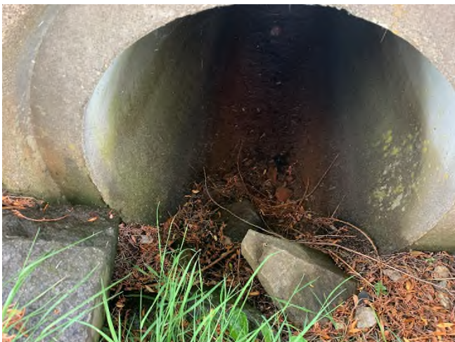
64 Gundalow – 2 (Drainage Course)
