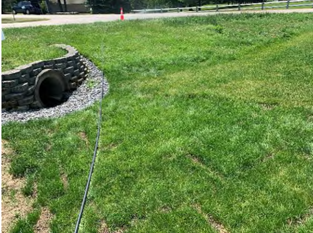
29 Gundalow -1 (Drainage Area)
