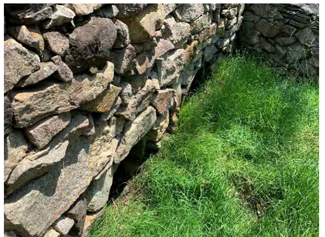
4 Brickyard Circle - 1 (Drainage Course)
