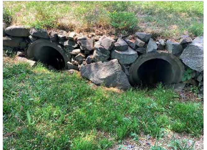
64 Gundalow -2 (Drainage Course)
