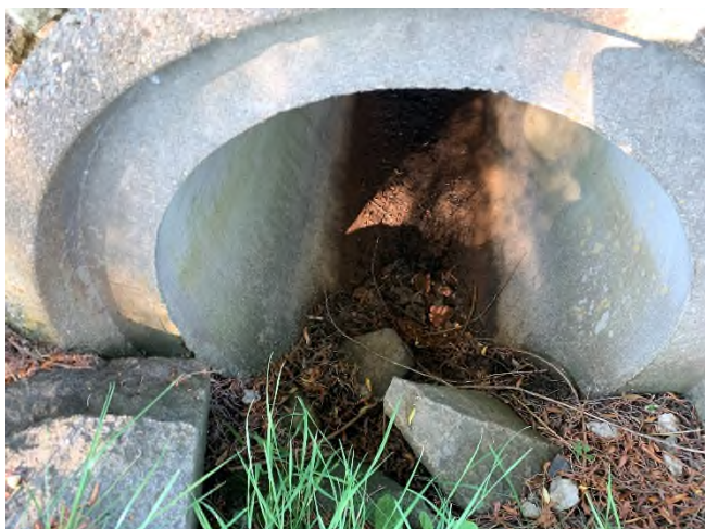
64 Gundalow - 2 (Drainage Course)
