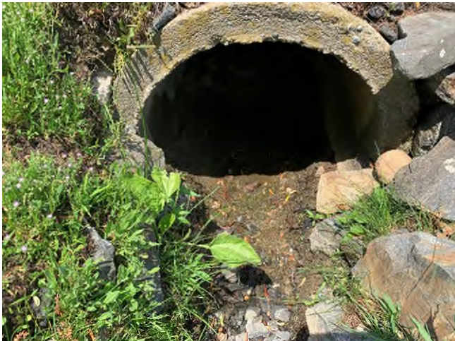
64 Gundalow - 1 (Drainage Course)
