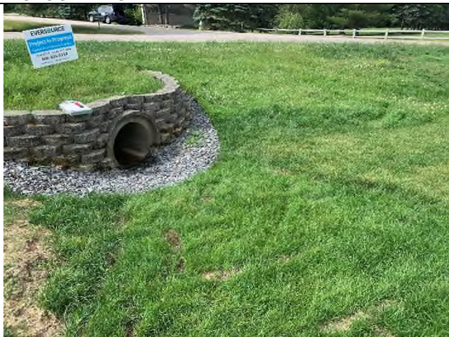
29 Gundalow -1 (Drainage Area)
