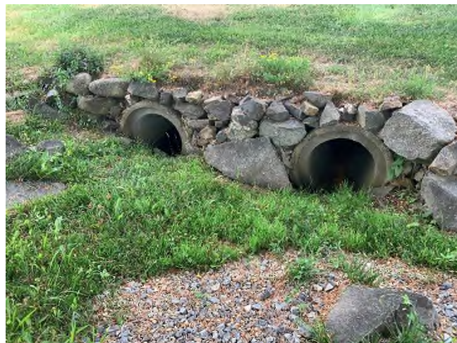
64 Gundalow -2 (Drainage Course)
