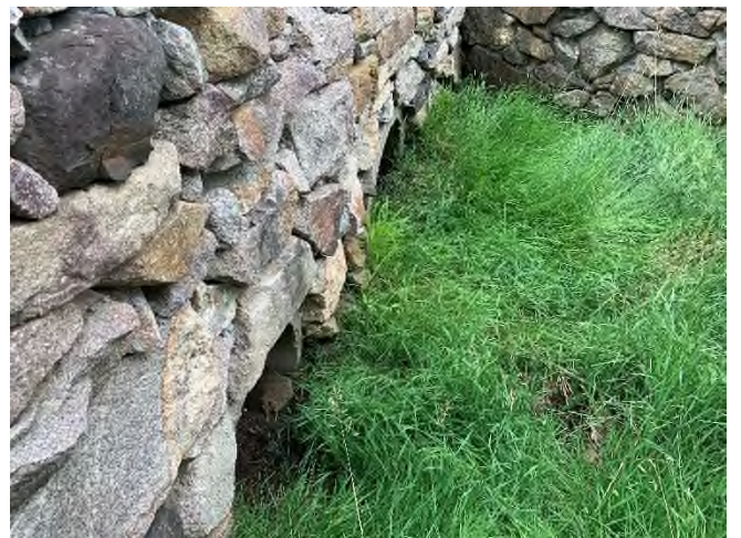
4 Brickyard Circle – 1 (Drainage Course)
