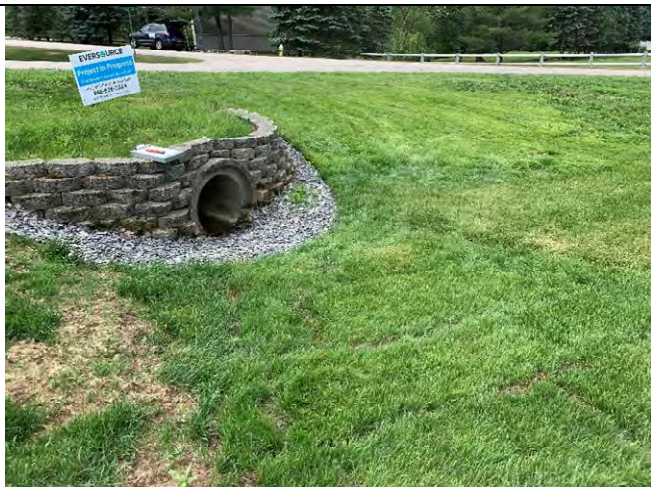
29 Gundalow -1 (Drainage Area)
