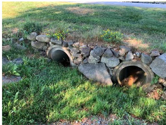
64 Gundalow -2 (Drainage Course)
