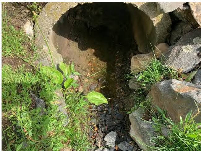
64 Gundalow - 1 (Drainage Course)
