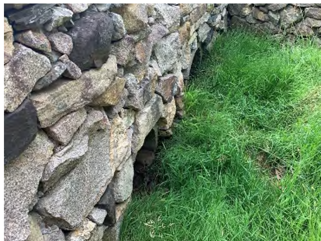
4 Brickyard Circle - 1 (Drainage Course)
