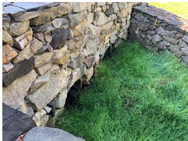
4 Brickyard Circle - 1 (Drainage Course)
