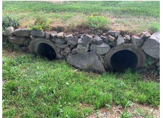
64 Gundalow -2 (Drainage Course)
