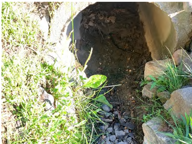
64 Gundalow - 1 (Drainage Course)
