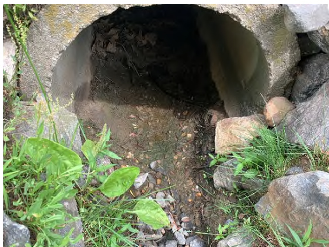
64 Gundalow - 1 (Drainage Course)
