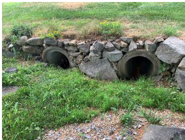
64 Gundalow -2 (Drainage Course)
