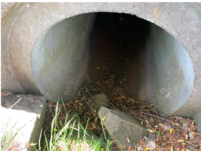
64 Gundalow - 2 (Drainage Course)
