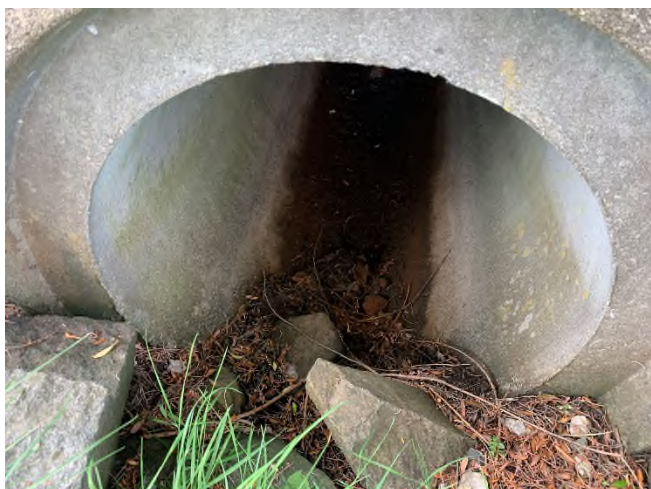
64 Gundalow - 2 (Drainage Course)
