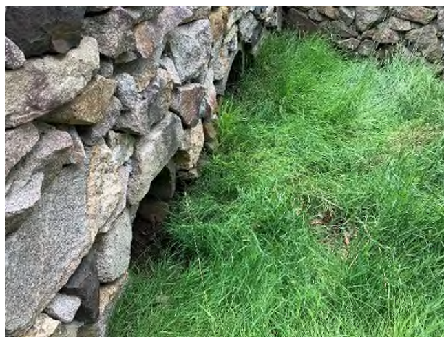
4 Brickyard Circle - 1 (Drainage Course)
