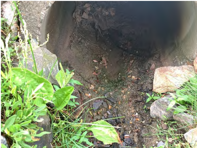
64 Gundalow – 1 (Drainage Course)
