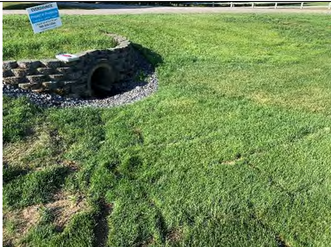
29 Gundalow -1 (Drainage Area)
