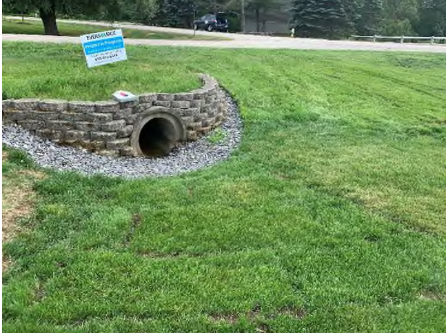
29 Gundalow -1 (Drainage Area)
